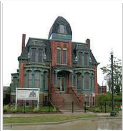
Historic restoration of the Second Empire style Frederick Butler House (1882), 8,400 square ft., at 291 Edmund Place in Brush Park (Woodward East), completed in 2006. [37]
