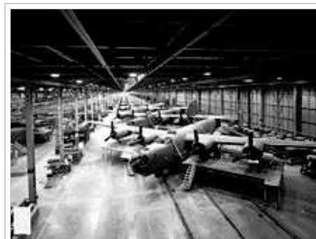
B-24s under construction at Ford's Willow Run line.
